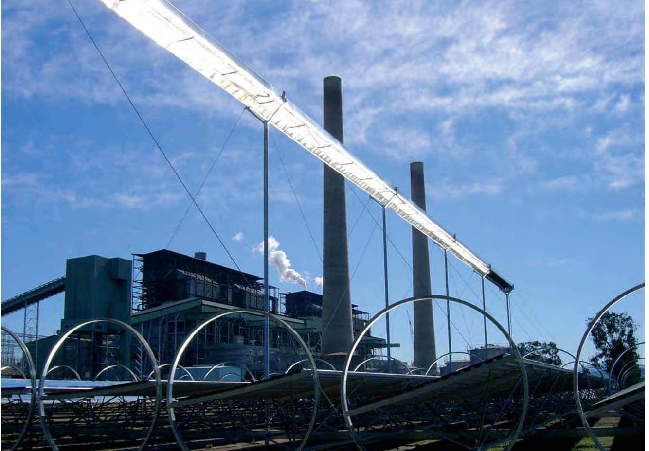
CS Energy's Kogan Creek Solar Boost project will use compact linear fresnel reflector technology at Liddell Power Station (Photo courtesy of AREVA Solar)
